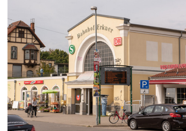
S-Bahnhof Erkner/suburban train station
